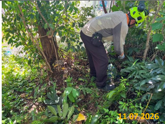
Removal of adjacent undersize trees within the protection zone
